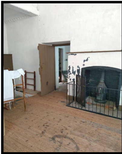
Inside the laundry
