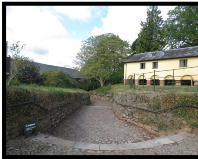
Cobbled path with handrails down to visitor reception
