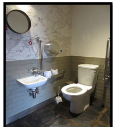
Accessible toilet by the Dairy café
