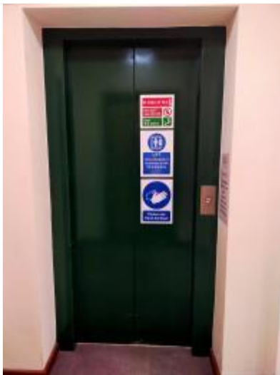
Main lift door from the first floor landing.
