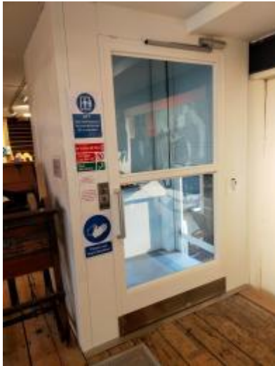
Lift door at ground level in the Goods Shed gallery.
