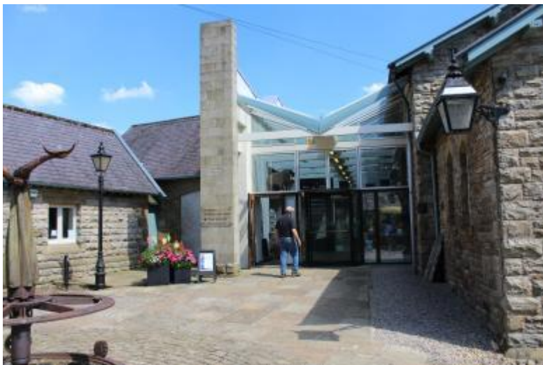
Museum entrance showing the slope up to the doors. The side door is to the left of the revolving door.
